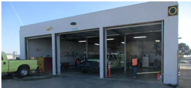
Airport Maintenance Facility, Airside View
