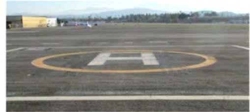
Helipad, Viewed from the South
