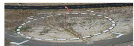
Wind Cone and Segmented Circle
